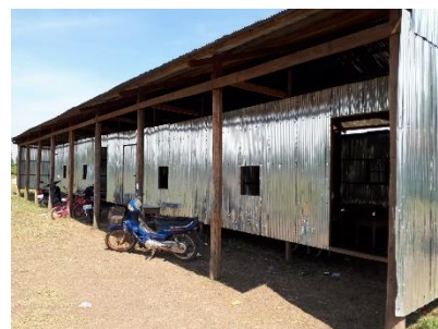
The temporary tin shack is sitting directly on dirt floor.
