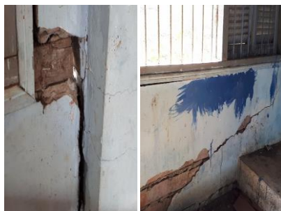
The vertical posts and walls are severely cracked and can collapse anytime.
